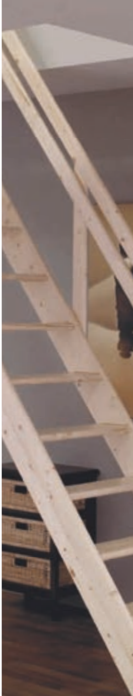
Stringer stairs made of wood
